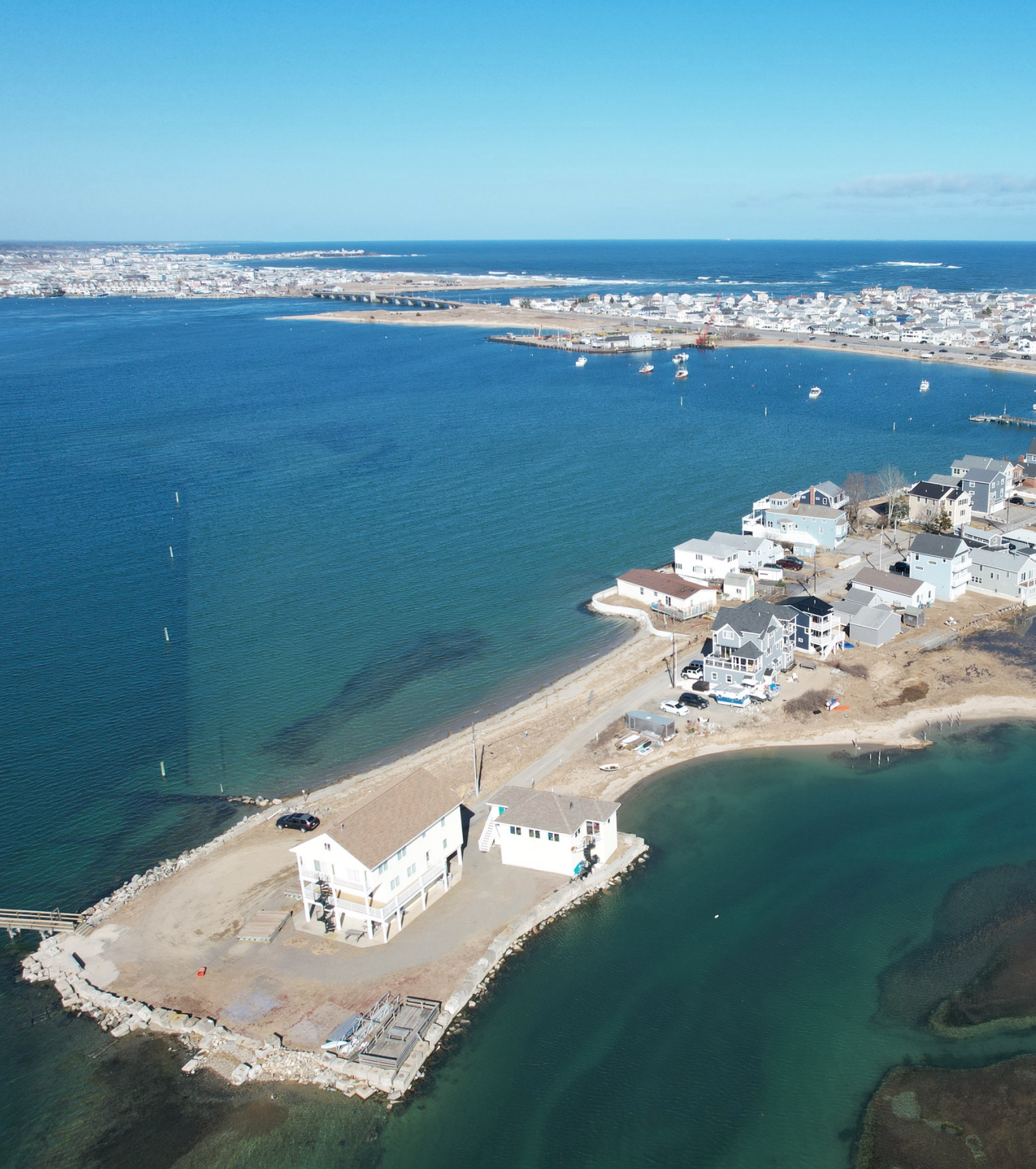
Image 21. River Street viewed from the southwest. Photo: Tom Morgan.
