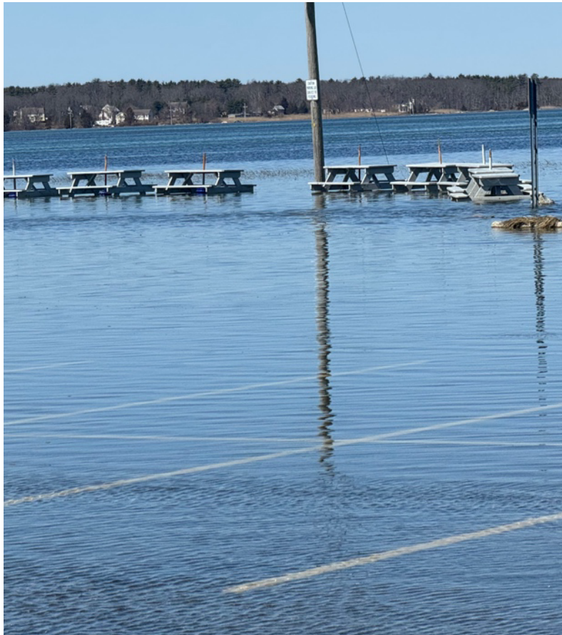
Image 20. High Tide Flooding along Route 286 on April 9, 2024. Photo: Tom Morgan
